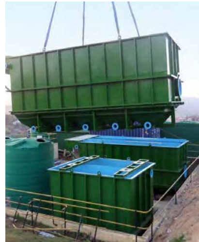
Steel or GRP Lamella Clarifiers
