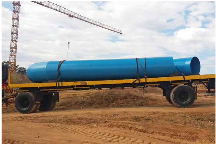
1000 mm with 700 & 800 mm branches Pipe item pipe item getting delivered at Rosetta WTW
